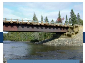
Less weight transferred to foundations when compared to other deck materials
